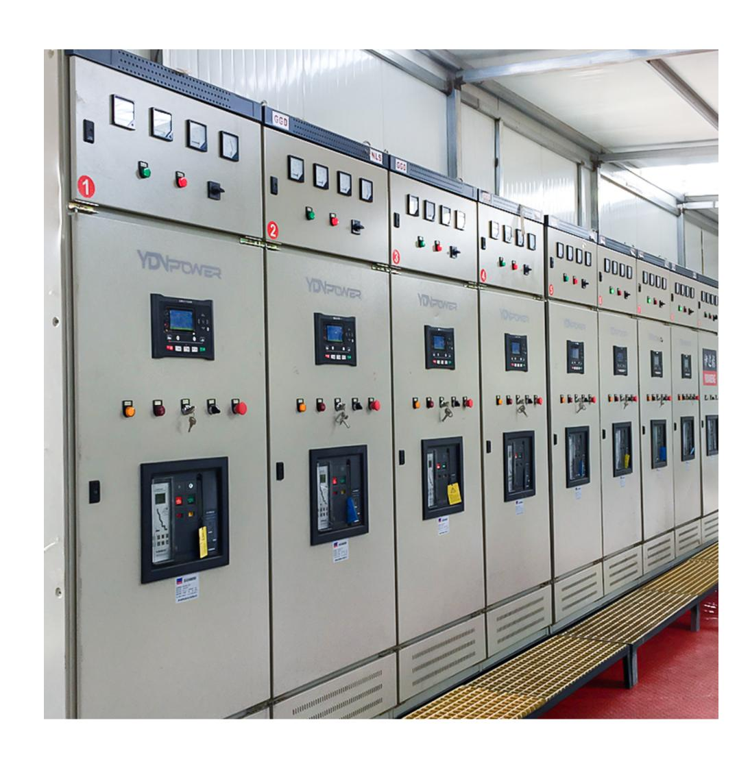
Sinopec's natural gas liquefaction project located in Yulin, Shaanxi province, uses 8\*250kW (total power 2MW) natural gas generating units, which operate alone to supply power to the compressor of the liquefaction plant.
